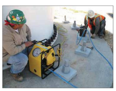
◀ In remote locations working off a generator the reliable Enerpac ZUTP1500 delivers the ultra high pressure needed for tensioning applications.
